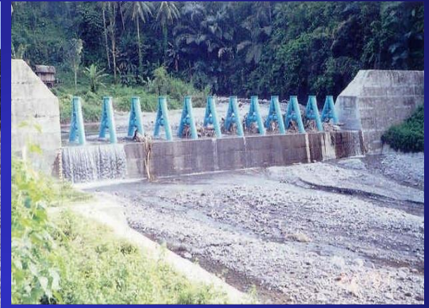
Anilao Slit-Type Sabo Dam
