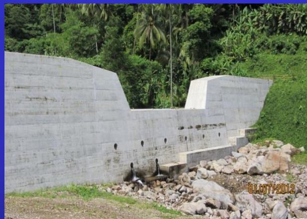
Camiguin Sabo Dam
