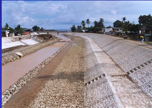
Ormoc Flood Mitigation Project
