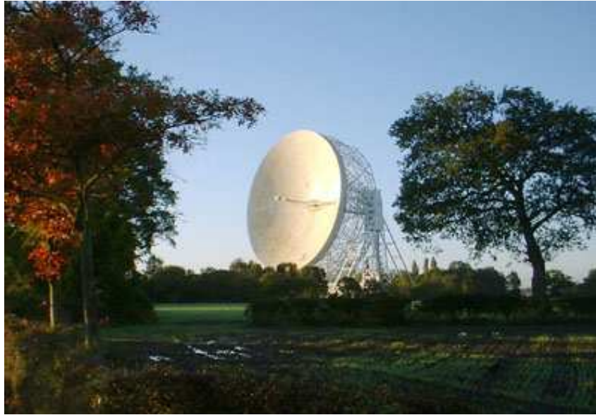
Figure 3.2 The Jodrell Bank antenna in the United Kingdom is 75 m in diameter.
