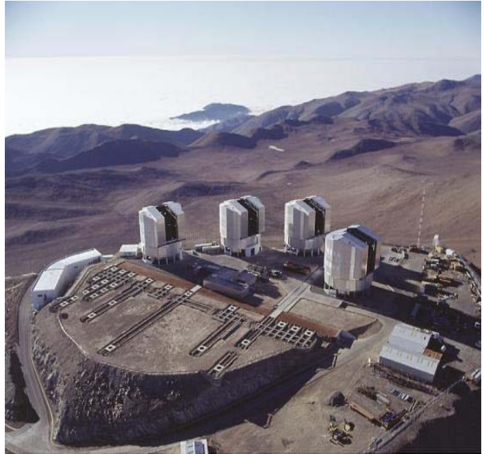
Figure 9.5 : The Very Large Telescope (VLT) is a set of four telescopes, each equipped with a 8m diameter mirror, located in La Silla (Chile) and operated by ESO, the European Southern Observatory. The telescopes can operate independently or in combined (interferometry) mode. The frequency covered ranges from near UV to IR (25 \mu m).
