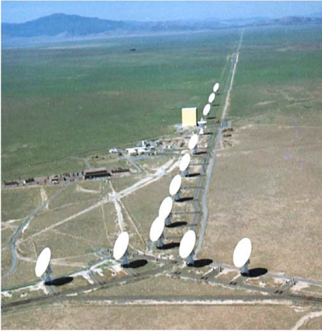
Figure 9.4 : The VLA (Very Large Array) is an interferometer made of 27 antennas arranged in the shape of a Y located in the US (New Mexico). Each antenna has a diameter of 25 m. They cover a frequency range between 74MHz and 50GHz. At 43GHz the resolution is 0.04 seconds of arc.
