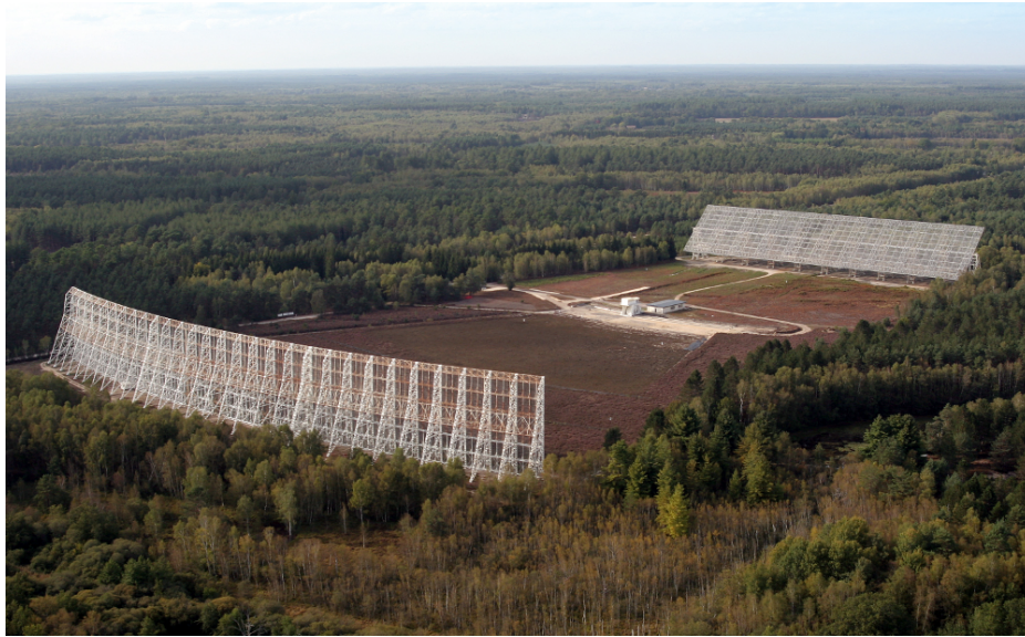
Figure 2.6: The Nançay (France) radio telescope. The tilting plane mirror in the background sends an image of the source to the fixed spherical mirror in the foreground. The mobile receiver system is visible between the two mirrors.
