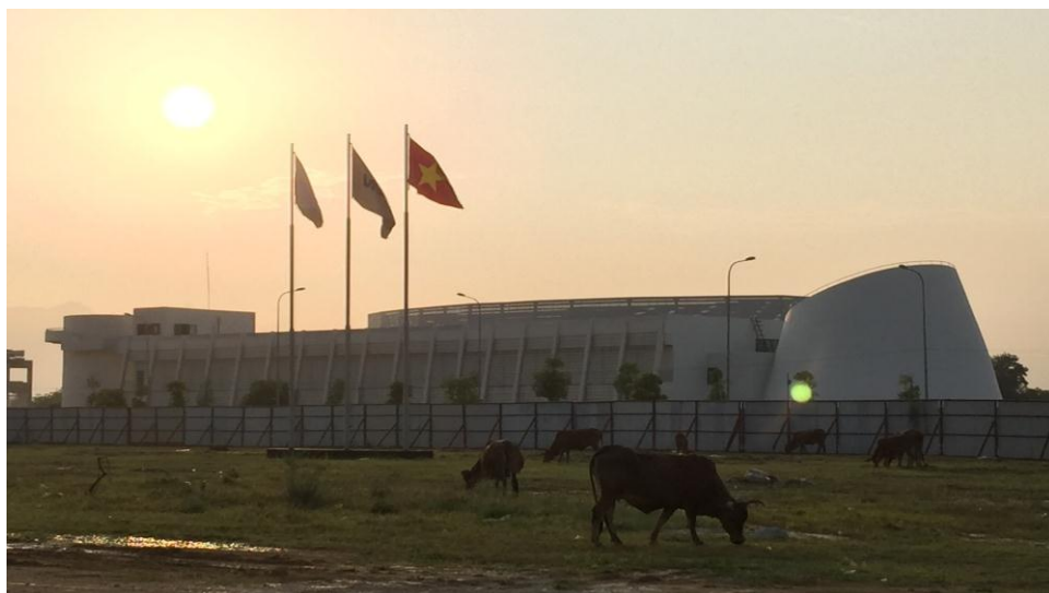
Part of the Hoa Lac Space Center seen from the back. The telescope building is on the left, waiting for its dome to be installed; the Planetarium is on the right; the Museum is in-between.
