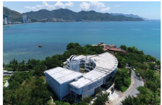
Nha Trang Observatory is located near the city in a beautiful site overlooking the sea. The buildings are shared between the Observatory and an oceanography institute.
