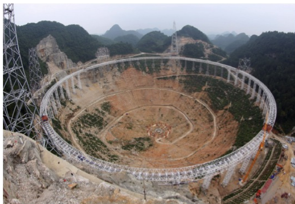
FAST: Status of the construction work, June 2014
