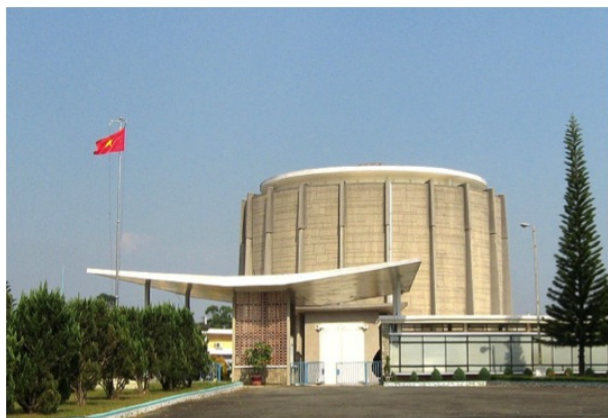
Da Lat research reactor building
