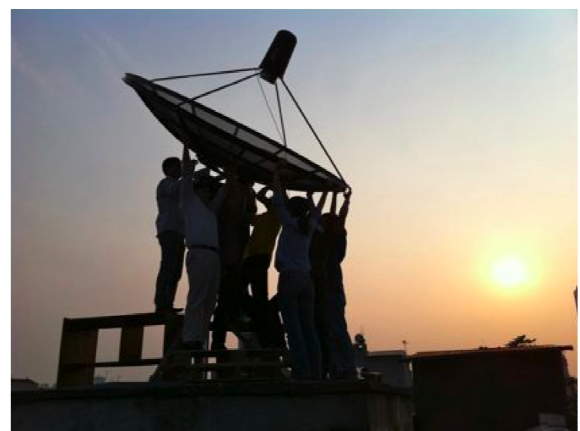
Installing the dish of the SRT on the VATLY roof
